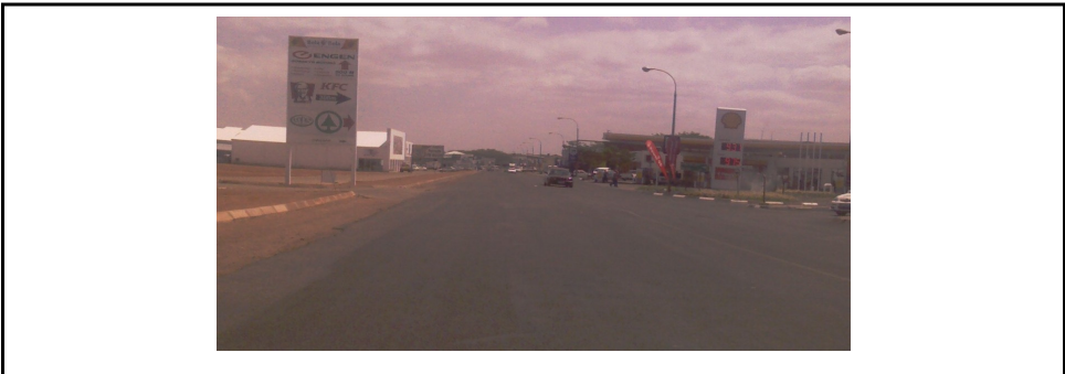
Photos 10: The condition of Potgtier Street after resealing
