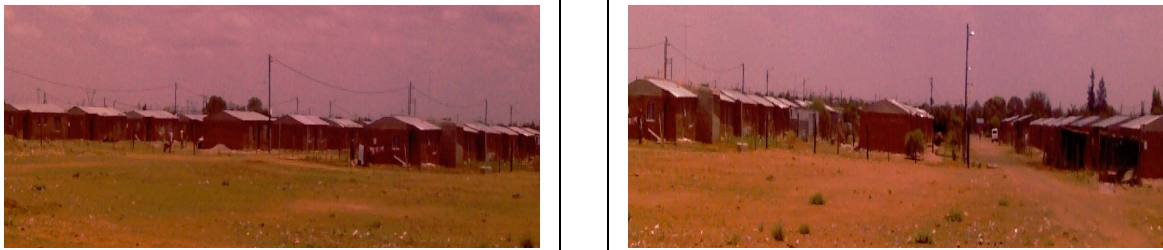
Photos 1 & 2: A side view of the 50 completed RDP units as part of the Youth Project in Bela Bela Township Extension 7
