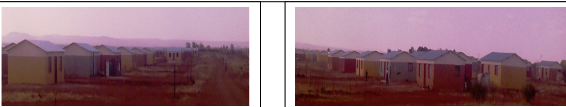
Photos 6 - 7: Side view (2) of Radium Low Cost (RDP) Housing Project
